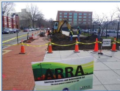
Figure 8: An impervious surface removal and tree planting project.
